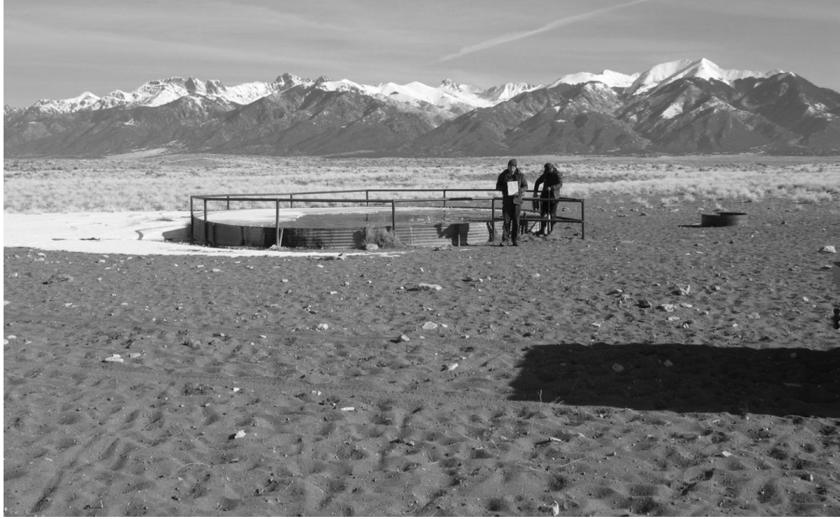
Figure 2.2 A capped artesian well site, prior to the study, comprised of a 5-cm steel pipe and the now empty water tank in the Great Sand Dunes National Park, Colorado, April 2010 (Photo by James Harte, NPS). Note the piosphere around the tank.
