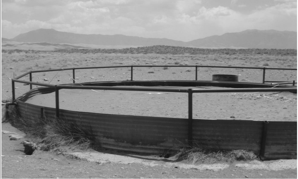
Figure 1.3 A typical capped artesian well site comprised of a 5-cm steel pipe and the now empty water tank in the Great Sand Dunes National Park, Colorado, 2011 (Photo by Sarah J. Garza).
