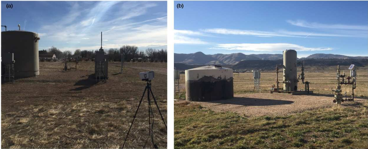
Figure 2.3: (a) Well pad 1 is a 10 m × 10 m wet gas production facility consisting of 1 wellhead, horizontal separator, and liquid storage tank. (b) Well pad 2 is a 10 m × 10 m dry gas production facility consisting of 1 wellhead, vertical separator, and liquid storage tank.
