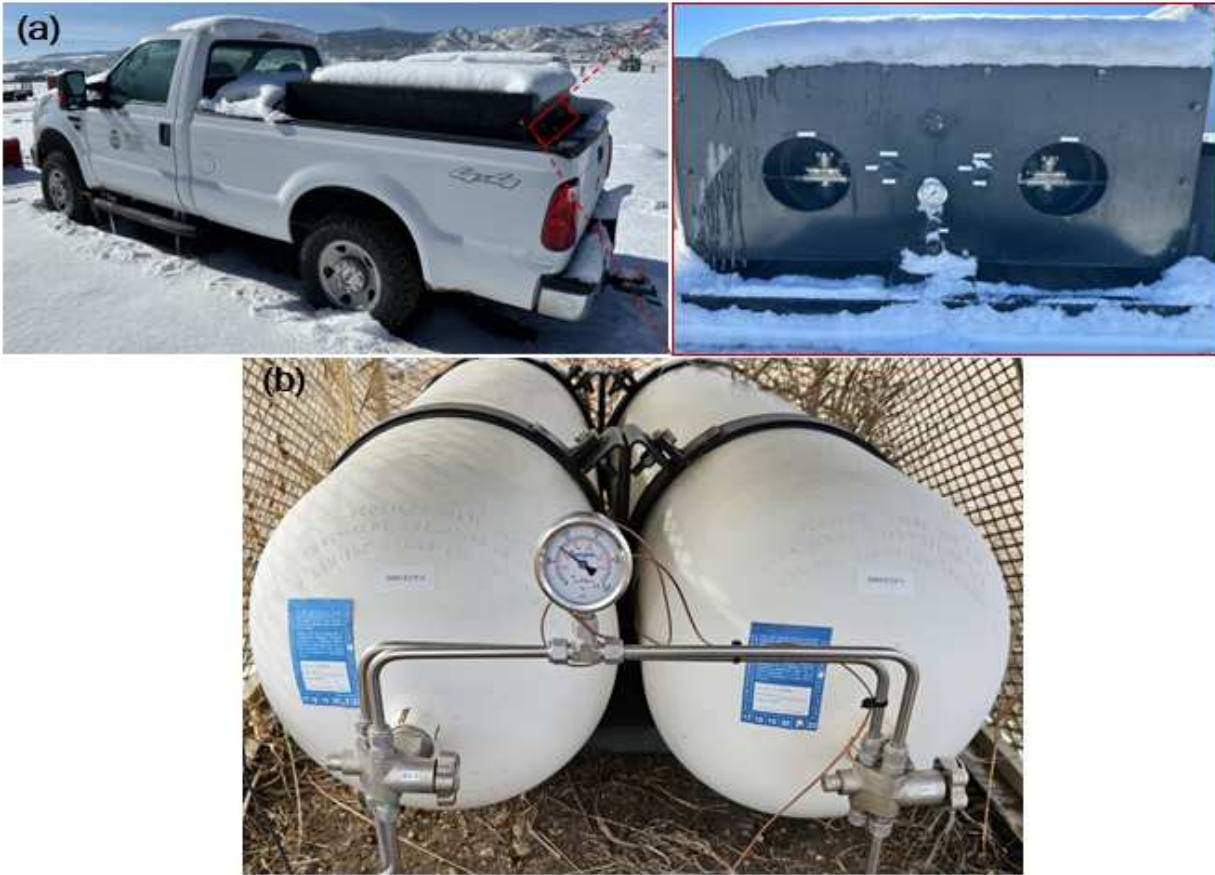
Figure 2.9: The top panel (a) shows the truck used for supplying compressed natural gas (CNG) to the onsite gas storage canisters/cylinders at METEC. The bottom panel (b) shows a set of the 290 liters, 3600 psi-rated steel canisters attached to each gas supply house at METEC, used for storing CNG.
