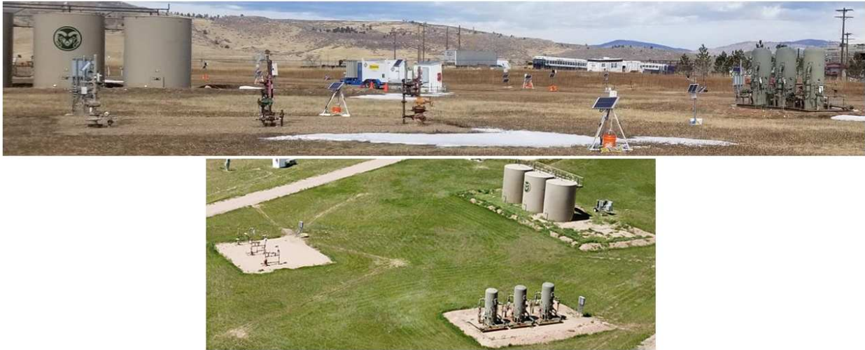
Figure 2.6: METEC pad 5 is a 60 m × 60 m production well pad consisting of 3 wellheads, 3 vertical separators, and 3 liquid storage tanks.
