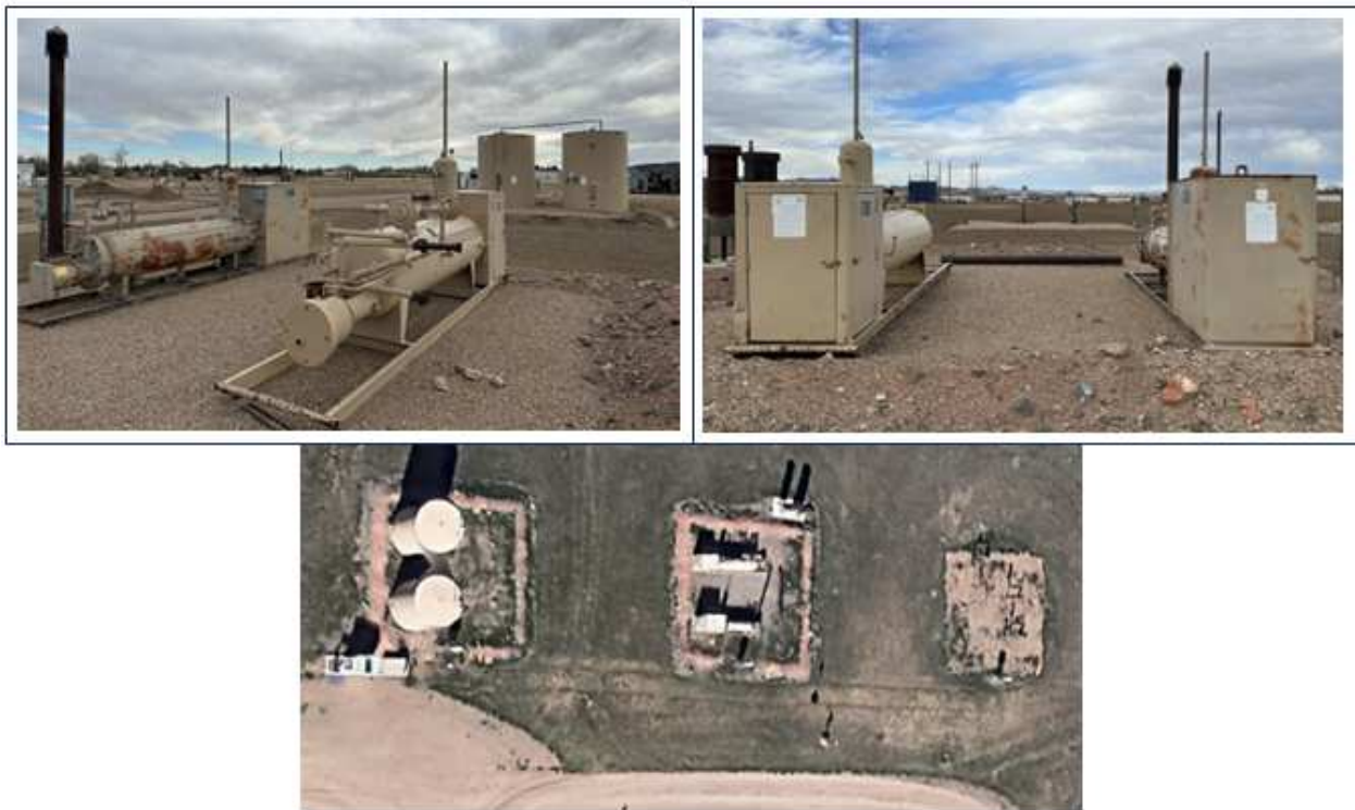
Figure 2.4: Well pad 3 is a 60 m × 10 m wet gas production facility consisting of 3 wellheads, 2 horizontal separators, and 2 liquid storage tanks.
