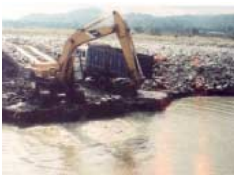
Photo 4. Channel excavation
