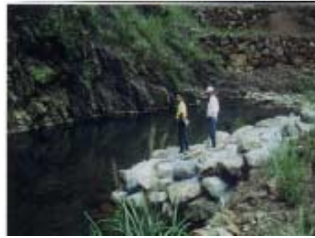
Photo 5. Concrete deflector with rock pavement
