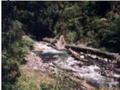
Photo 10. Dam No.4 recent condition (Oct., 2001)
