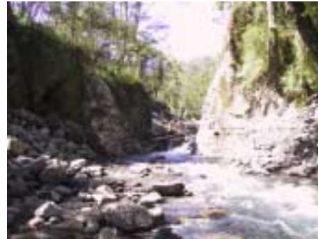
Photo 14. Dam No.2 recent condition (Oct., 2001)
