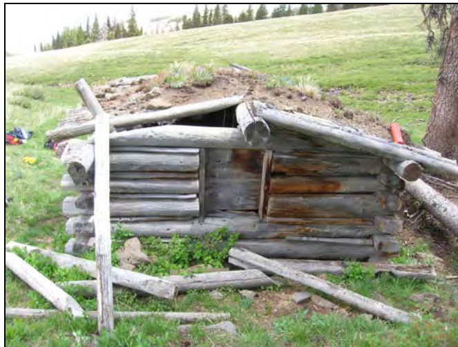
Figure 4.5. The west elevation of Webster Creek Cabin
