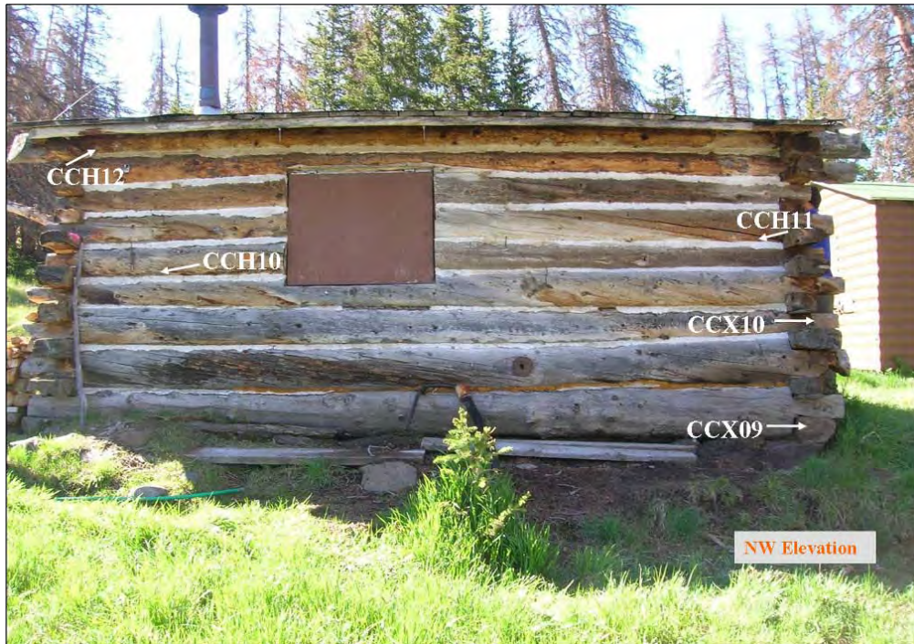
Figure 4.4. Sample CCH10, collected from the 5 th course, northwest-facing elevation of the main cabin at the Jack Creek Cow Camp. The location of the sample is to the left of the shuttered window.
