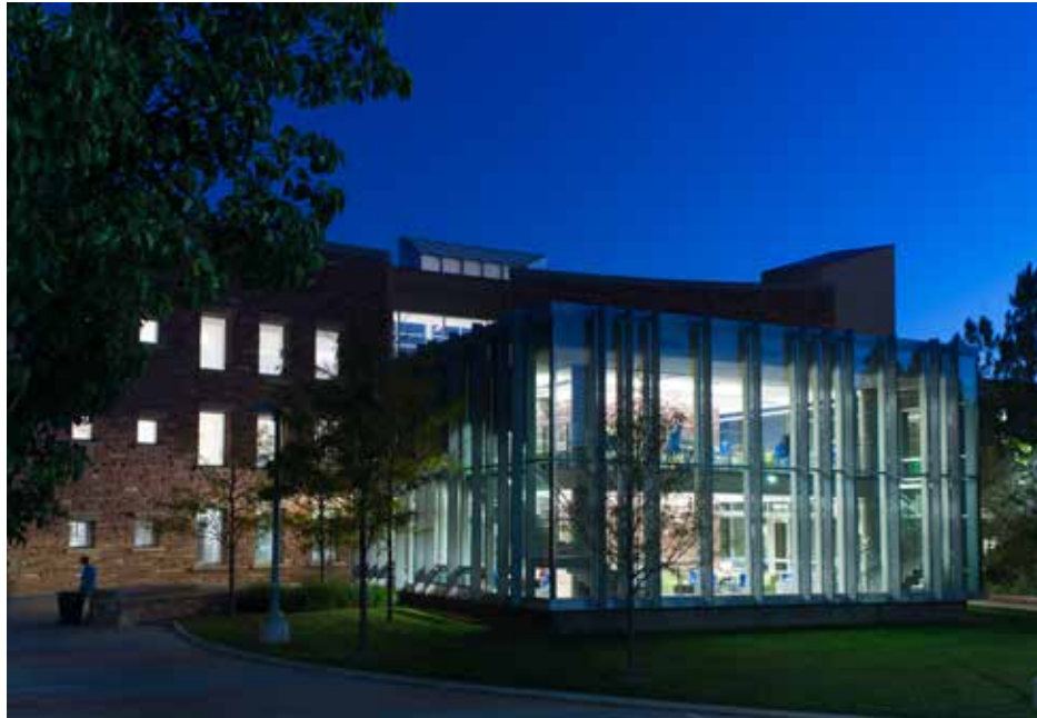
In 2010, electrochromic glass, commonly referred to as smart glass, was installed in the Study Cube as a part of CSU's sustainability efforts.
