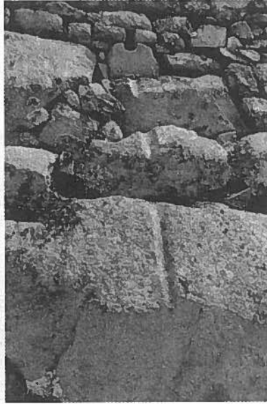
Fig. 14. An example of an Urban Drainage outlet (upper center) with a vertical drop channel cut into the stone wall rocks below the outlet.
