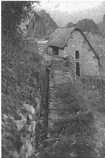
Fig. 7. Inca domestic water canal entering the Agricultural Sector. Cut granite stones forming the right bank contribute to hydraulic efficiency. The two-story building was for grain storage.
