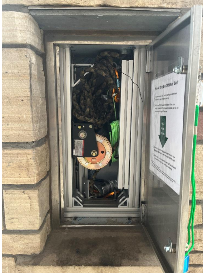
Figure 7: Completed system installed in box
