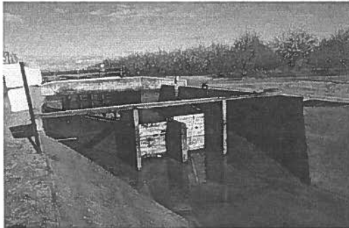
Figure 4 - Long Crested Weir
