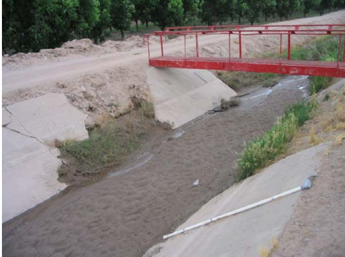
Figure 13. Concrete lined section of the Del Rio Lateral
