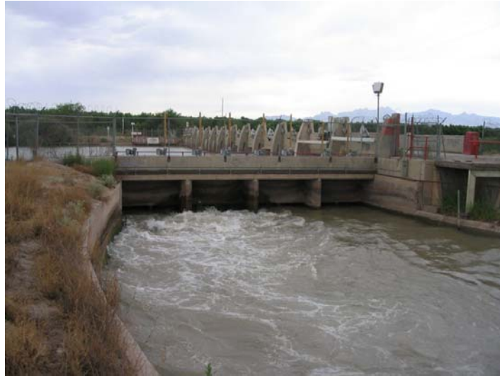
Figure 11. Turbulence downstream of the head gates on the West Side Canal
