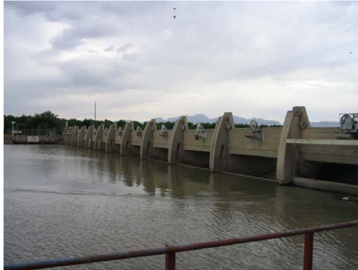
Figure 9. Upstream face of the Mesilla Diversion Dam
