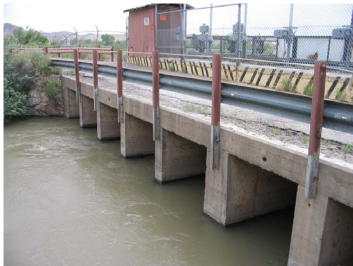
Figure 7. Submerged sluice gates at the head of the Leasburg Canal
