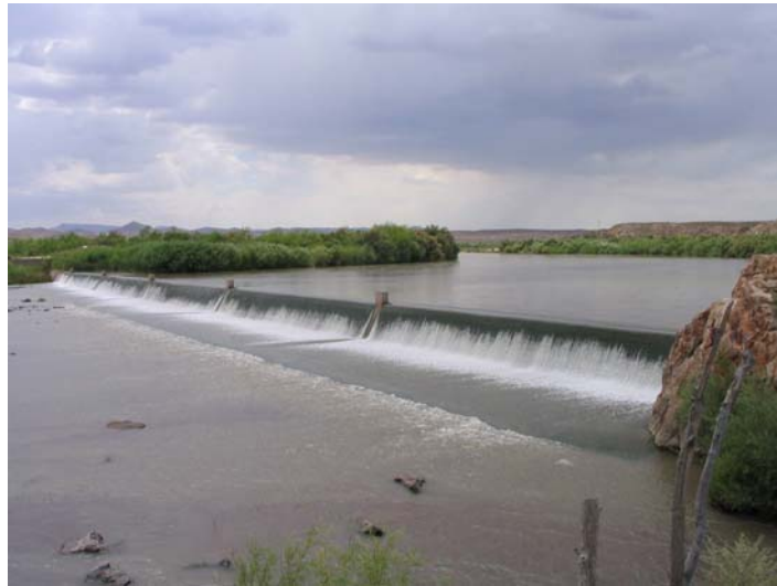
Figure 6. Leasburg Diversion Dam
