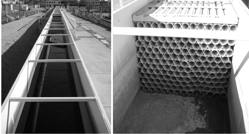
Figure 3. Cal Poly flume, looking downstream (left) and honeycomb flow conditioner (right)
