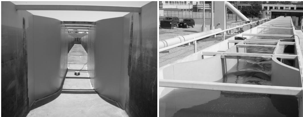
Figure 4. Subcritical contraction and SonTek-SW installed in the Cal Poly ITRC flume.
