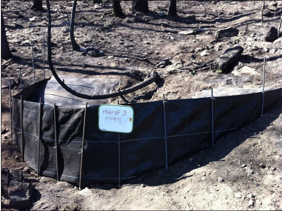
Figure 2.4: Sediment fence in upper Hill Gulch, installed 8 Sept 2012.
