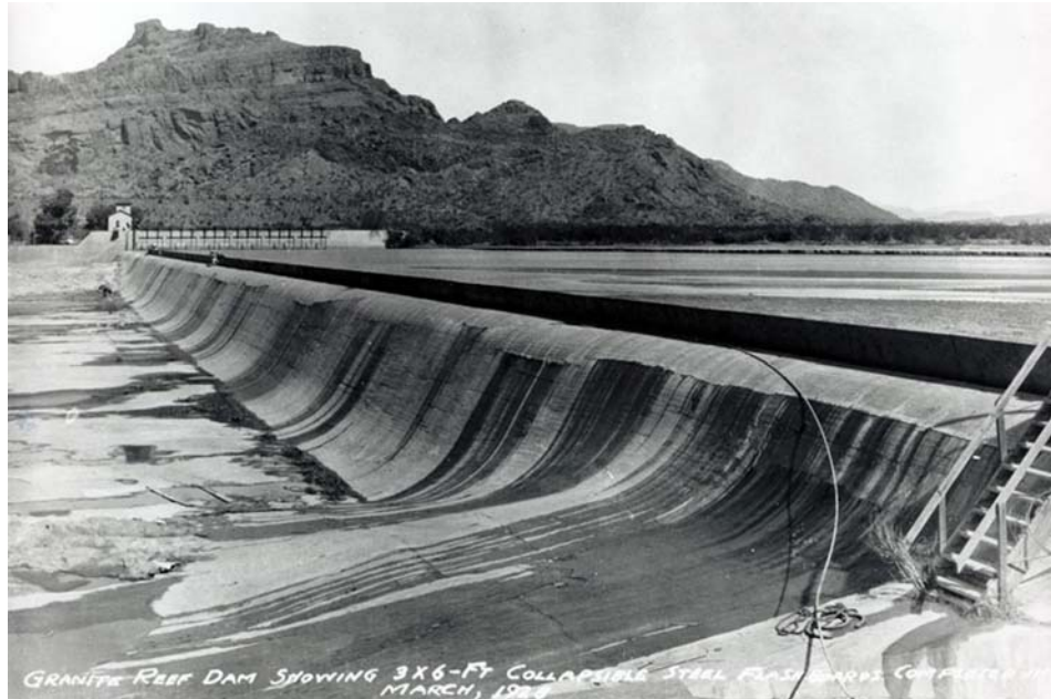
Image 2. Granite Reef Diversion Dam.
