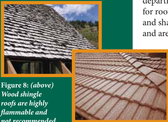
Figure 9: (above right) Class A roofing materials including tile, clay, concrete, slate and asphalt shingles are fire-resistant options. Photo: CSFS
